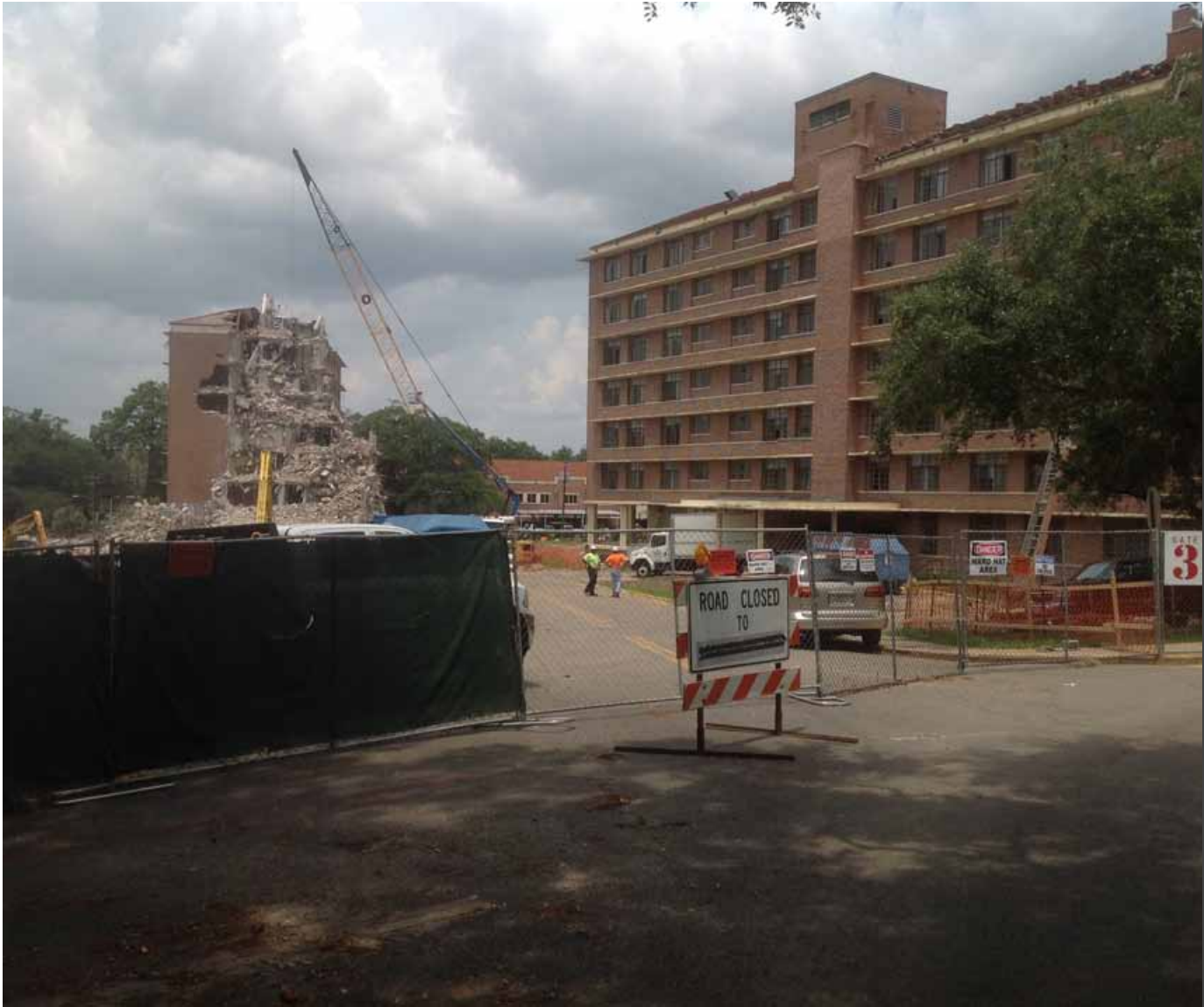
The original Dorman Residence Hall is nearly demolished and they will then demolish Deviney Residence Hall
