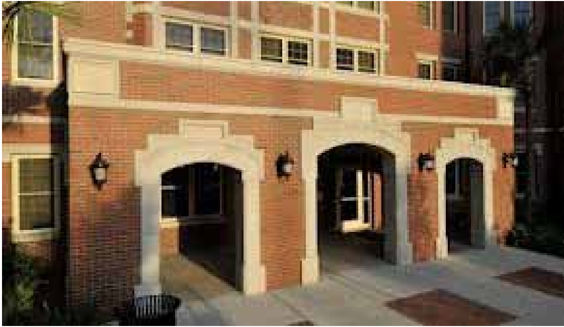
Front Entrance to Traditions Hall
